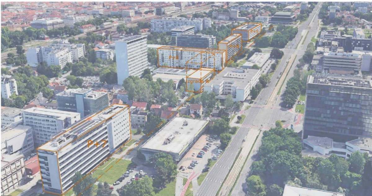
Figure 2. Second row of buildings in Vukovarska Street
